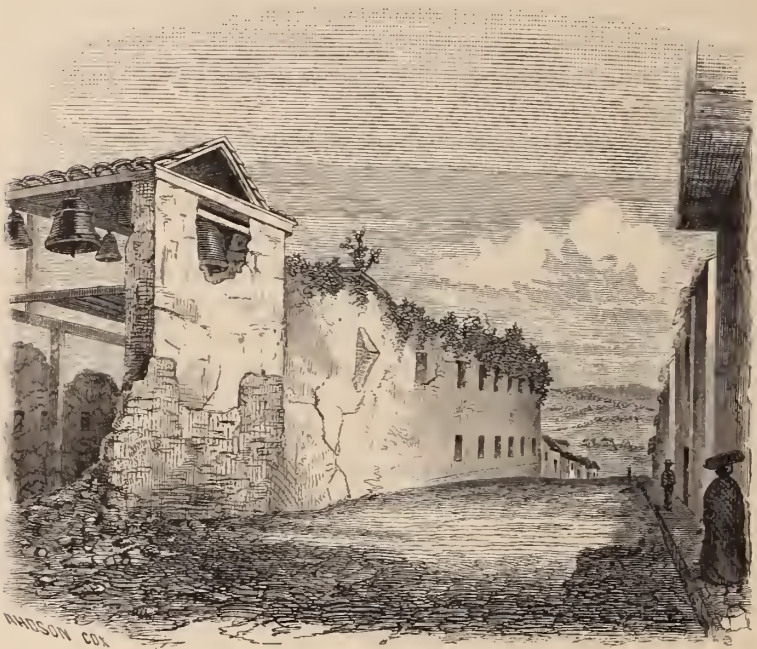
WHAT THE EARTHQUAKES LEFT
